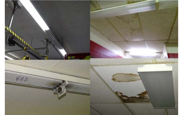
Central Fire Ceiling and Lighting
